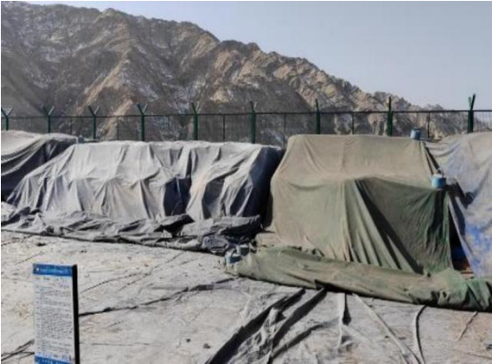
物料篷布苫盖
