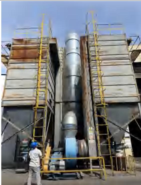
压铸工序脉冲除尘
