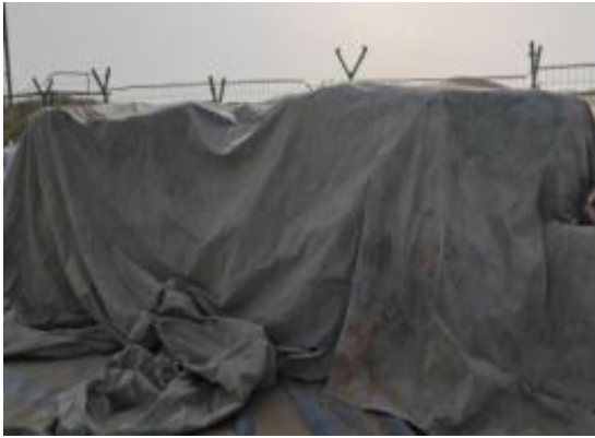
物料篷布苫盖
